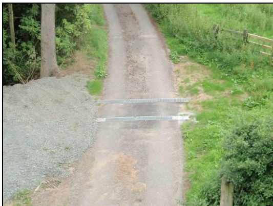
Figure 8 - Crawley Farm Road Surface Water Strip Drains
