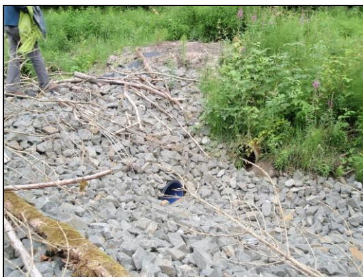
Figure 4a – Storage embankment with 300mm diameter outlet pipe
