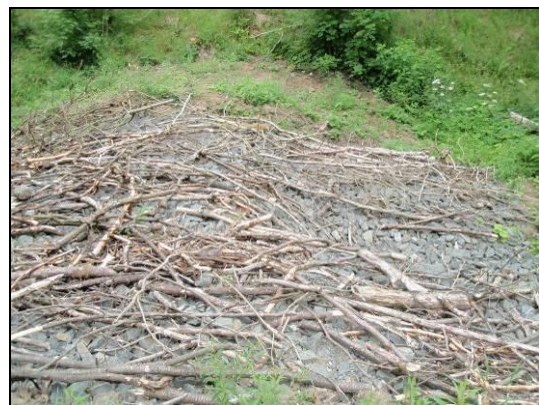
Figure 4b – Armoured embankment crest
