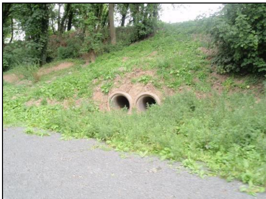
Figure 11 – New Railway Embankment Culverts
